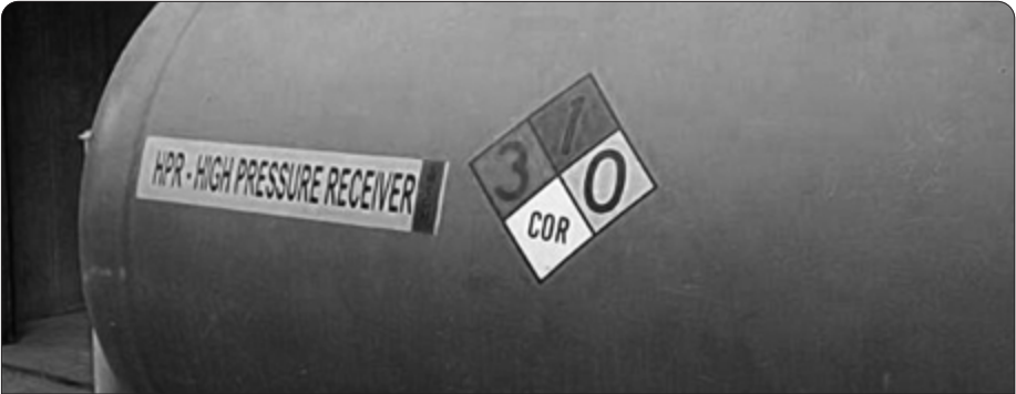
Image 83. NFPA:704 Diamond. The tank contains a chemically stable, extremely corrosive chemical that is non-flammable at room temperature.
